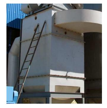
assures uniform gas distribution and proper flow to each individual collecting tube for maximum design efficiency. The cyclone housing is constructed from steel plating, and contains doors for inspection and cleaning. The inand outlets are flanged. The frame is constructed from stable angle profiles, and can also be delivered with non-standard heights if necessary.
